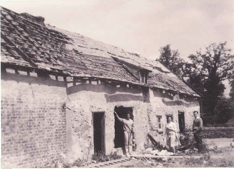
Left. The old cottages, where 'Siesta' now stands, being demolished in 1959.
